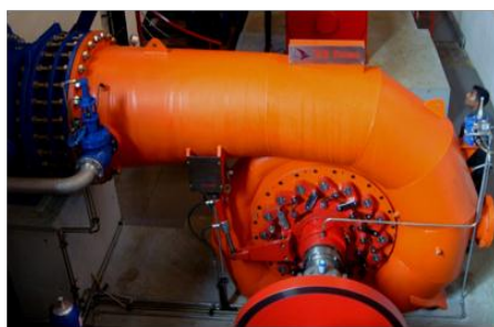
Locally manufactured hydro turbine
